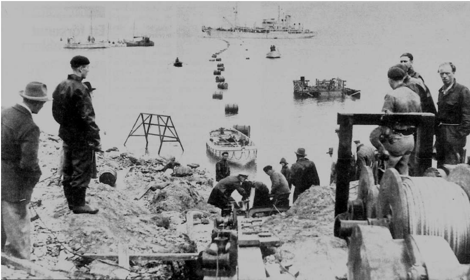
Figure 1.1: During the summer 1953, the cable of the first commercial HVDC link is drawn ashore south of Visby on the island of Gotland, Sweden (courtesy of ABB).
